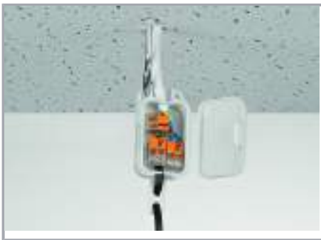
Pendant light connection in a suspended ceiling
